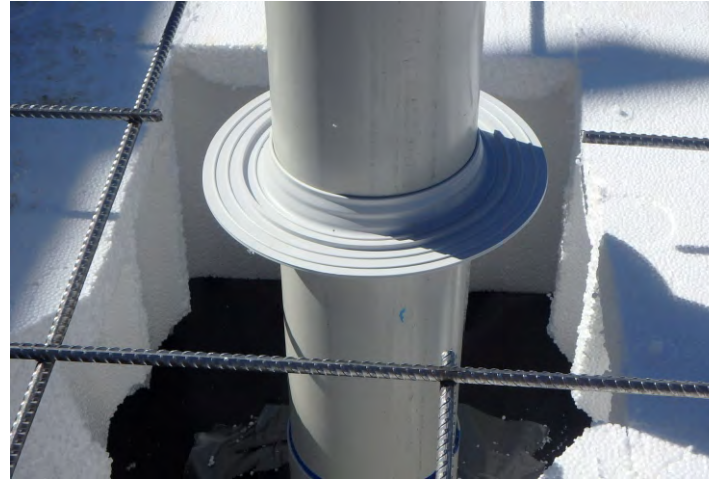
Termstop Termite collars key strongly into the concrete to block termite access.
