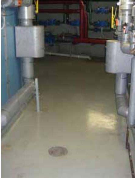
**Computer or Server Rooms** - Floor wastes or tundishes in these areas require an easy solution to ensure odours do not make their way into these rooms. As no water points are allowable, evaporation is an issue, creating a dry waste, which increases odours.
